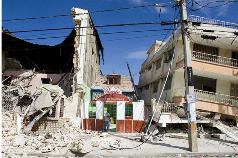
Earthquake damage in Haiti – people lived here before the earthquake
